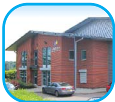
Easter Court Lasertech Head Office located in Warrington.
